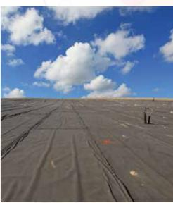
TerraTextile® is a specially made technical textile, either woven or non-woven. They offer excellent strength and hydraulic characteristics; and cater for a wide range of applications. Woven TerraTextile® is used for soil reinforcement, separation and filtration, secondary reinforcement, erosion control, ground stabilisation, silt fence etc. Non-woven TerraTextile® is very popular in applications such as filtration, separation, sub-surface drainage and transmission erosion control.
