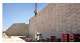
Composite Earth® technology adopts primary and secondary soil reinforcement systems for the design of Reinforced Earth® retaining walls. It aims to control the lateral deformation of the facing during construction and operation, including during seismic events. This is an effective way to design and construct tall and critical structures.
