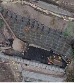
**Shored MSE®** technique allows building of earth retention structures connecting existing profiles stabilized by soil nails and/ or anchors. It is a useful technique for construction of benches and for road widening projects with limited available space, and activates the best optimisation between cut and fill requirements.
