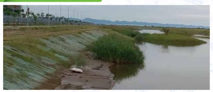
TerraGreen® is a custom designed erosion control mat / blanket useful for protecting dry and intermittently wet and erodible slopes. TerraGreen® as a stand-alone technique or mixed with other solutions like TerraNail® or TerraAnchor™ and high-tensile steel netting is often used to mitigate low to medium grade surface erosions and soil slips and slides.
