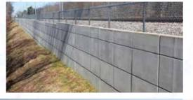
The **T-Wall**® system is a precast modular gravity type reinforced concrete retaining wall system. It is most suited for railway load supporting structures and construction of submerged retaining structures. The **T-Wall**® system decreases in stem length course by course – reducing materials, excavation and backfill as compared to other wall systems.
