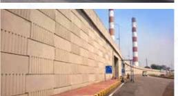
Reinforced Earth® structures combine engineered backfill with steel or synthetic tensile reinforcement and a modular concrete facing system. This ideal combination creates a durable and resilient earth retention structure. With **Reinforced Earth®** structures we can create several attractive architectural finishes.
