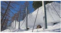
**Avalanche Barrier** systems are designed on a site-to-site basis to protect infrastructure, utilities, buildings, reforestation, and lives from avalanches. Snow nets, snow rakes and steel snow bridges are installed in the initiation zones to prevent avalanches from forming. Static defense structures, snow catchment fences/ barriers are used which effectively reduces the run-out length of an avalanche.
