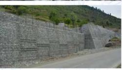
Reinforced soil slopes (RSS) are an extension of the Reinforced Earth® technique. This structures are designed and built to retain with a face inclination of between 45° and 70°. ArmaGreen is the name of our vegetated facing solution, while ArmaStone is the name when we use a mineral facing.
