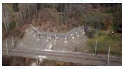
The Reinforced Earth Company offers engineered solutions to protect infrastructure, and assets from debris flows and debris floods. The threat of climate change raising the global temperatures, potentially causes a change in weather patterns, thawing of permafrost areas, increasing wildfires, debris flows, and shallow landslide activity. The use of flexible-net barriers can be an efficient alternative to the other traditional and costly mitigation measures such as dams and other rigid barriers.
