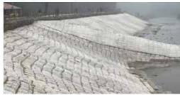
**TechRevetment®** is a pre-engineered factory costumed grouted mattress system used for permanent erosion protection works. This technology is used to protect embankments, protect bridge abutments against scour, for bed protection of major rivers and waterways, and for shoreline protection. This system can be installed at rapid speed and under water without the need for dewatering.
