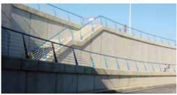
**TechWall®** precast retaining walls and abutments are effective solutions when a standard footing is used or when site conditions rule out the use of Reinforced Earth® structures. **TechWall®** is developed as an engineered product with low lifecycle costs and long- term performance, which helps minimize overall construction duration and reduces site works.
