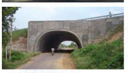
**TechSpan®** is a one of the most reliable, cost effective precast concrete arch systems available for cut 'n' cover structures. It is widely used in the construction of bridges, underpasses, conveyance and reclaim tunnels, portals, ammunition storage bunkers and rockfall sheds and shelters. Typically, 15-20 linear meters of **TechSpan®** can be installed in one work shift.
