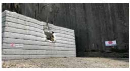
**TerraBund**® is a Terre Armée protection bund. It is a gravity structure built using soil reinforcement and flexible or semi-rigid facing systems. It is a passive protection system used typically as a geo-hazard solution against rockfalls, avalanches, debris flow and mud slides. TerraBund® can withstand more than 8000kJ of impact energy in the event of landslide or rockfall.
