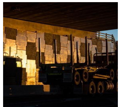
Main picture and above: TerraClass® true abutment walls at the ETA over Broadlands Rd Bridge
