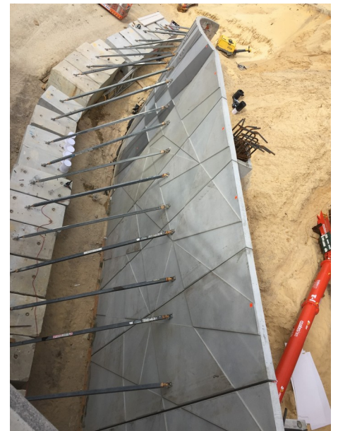
New abutments panels installed and relocated wingwalls in place
