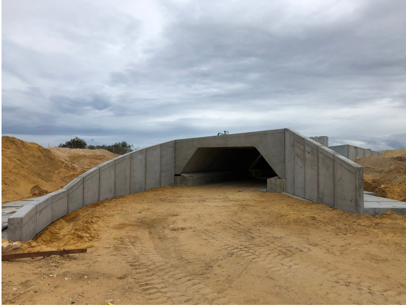
Trapezoid arch with spandrel and wingwalls
