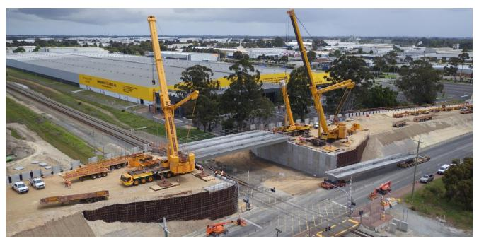
**Above:** Reinforced Earth® abutment walls and temporary wire walls applied to enable staged works. Seen here during the bridge beam install – photo courtesy of MRWA.
