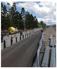
Main picture: Reinforced Earth® wall during construction Above first picture: Reckli® 2/49 Saale panel finish Above second picture: Placing backfill along rear of Reinforced Earth® wall
