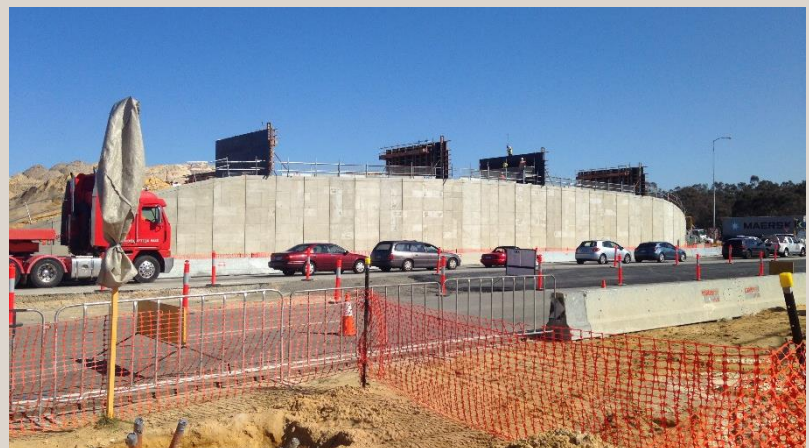
Above: Abutment wall at Malaga Drive Interchange during Construction
