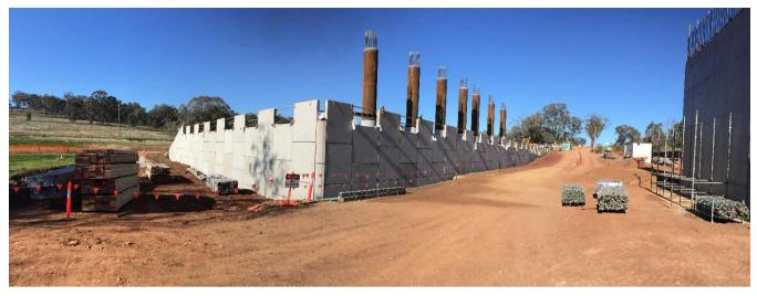
Above: Construction of the Reinforced Earth® bridge abutment walls begin.
