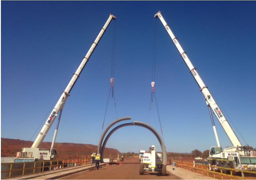
Left: Installation of the TechSpan® arches by RECO Above: TerraMet® Head and Wing Walls Below Left: Completion of TechSpan® Tunnel
