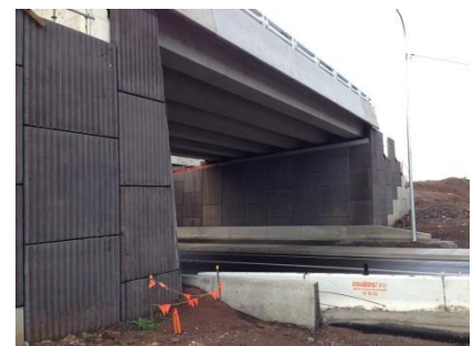
Main Picture: Reinforced Earth® Vertical Ribbed Panel Finish
