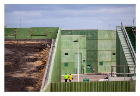
our regular visits to the construction site. With regard to the irregular sizing required for some of the walls, moulds for the TerraPlus® panels were specifically prepared to undertake the job, which led to a smooth transition from design to construction. This also meant that elements arrived ready for installation, and fast construction saved site costs.
