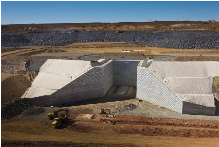
Left and above: One of RECO's completed TerraMet® dump walls.
