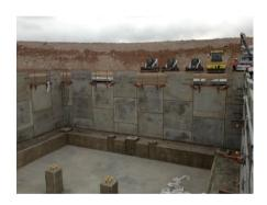
Main picture: TerraPlus® Dump walls near completion. Photograph courtesy of Retaining Solutions Pty Ltd Above first picture: Placement of the galvanized steel reinforcement strips. Above second picture: The slot arrangement at the centre of the dump walls.
