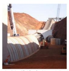
Installation of TechSpan® reclaim tunnel with a variable vertical alignment of up to 10% grade adding significantly to the design complexity and requiring wider arch units to ensure longitudinal arch stability.
