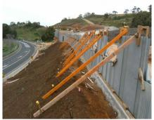
Left: TerraPlus® Reinforced Earth™ walls at the Pacific Highway Upgrade - Ballina Bypass. Above: Construction of the Reinforced Earth™ walls, Ballina, NSW.
