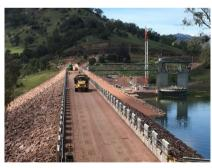
Main: View of the completed Reinforced Earth® upstream wall.
