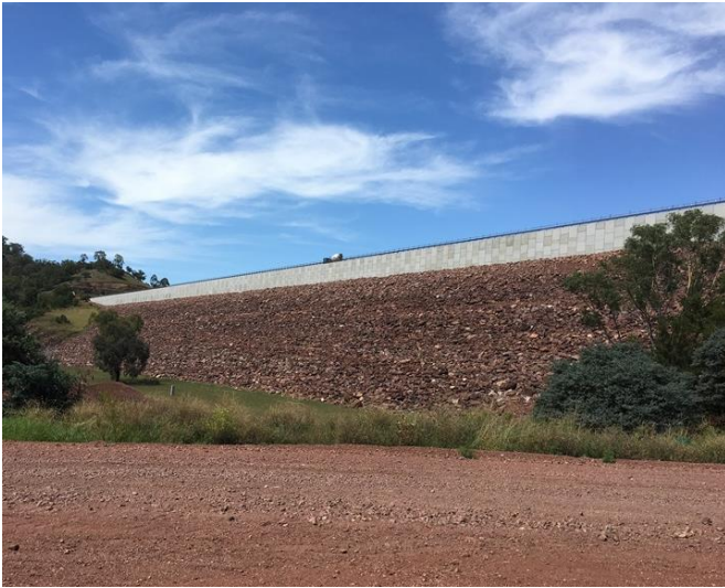
Above Left: View of the Reinforced Earth® downstream wall
