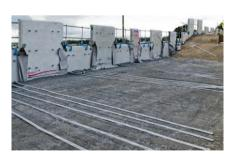
Main & Top: Horizontal rib panel finish. Above: REhas® galvanized steel reinforcing strips are unmatched for structural capacity and reliability.
