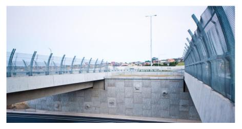
RECO worked closely with project architects and sculptors running through several design iterations during the progressive development of the exact panel finish required by the RTA and Fulton Hogan. The end result was two individual shell patterns and one Shellharbour Council emblem itself.
