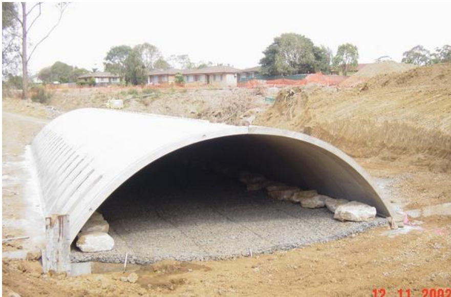
Left: The 33 metre arch structure is completed awaiting installation of headwalls. Stones located at the base of the arch within the waterway to minimise scouring of concrete. Above: Construction of TerraClass® wing walls. Note vertical rib architectural finish.
