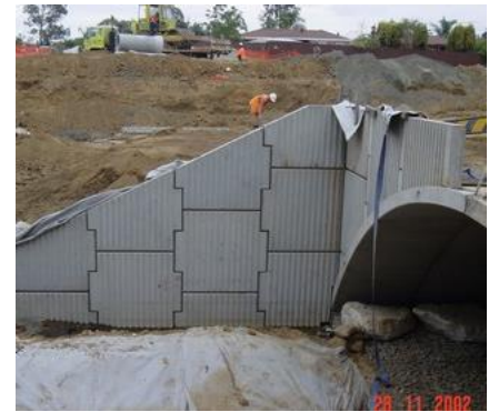
Left: The 33 metre arch structure is completed awaiting installation of headwalls. Stones located at the base of the arch within the waterway to minimise scouring of concrete. Above: Construction of TerraClass® wing walls. Note vertical rib architectural finish.
