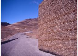
Main picture and above: Reinforced Earth® retaining walls, with TerraTrel® wire mesh facing panels, at the Cairnmuir Slide. Cromwell Gorge - Central Otago,
