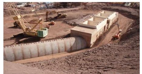
Main Picture: - TechSpan® construction in the middle of a very congested, fully operational, Tom Price mine facility
