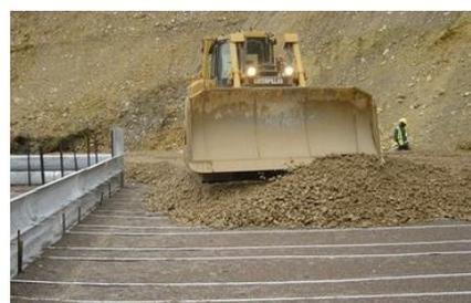
Main Picture: Construction of TerraMet® dump structure begins. Note panels and strips stockpiled on site, and grader and bulldozer spreading and compacting backfill, respectively.
