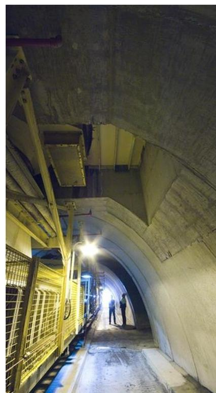
Main Picture: The TechSpan® reclaim tunnel is designed for a coal stockpile height of almost 30 meters. However, the more significant challenge for RECO's design team is that the shape and location of the stockpile changes continuously, generating unbalanced loading onto the tunnel below.
