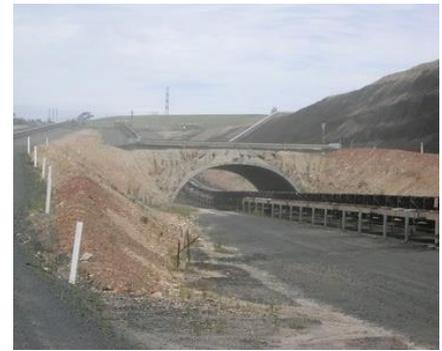
Left: Two of the Three Hazelwood Mine Conveyor TechSpan® Arches
