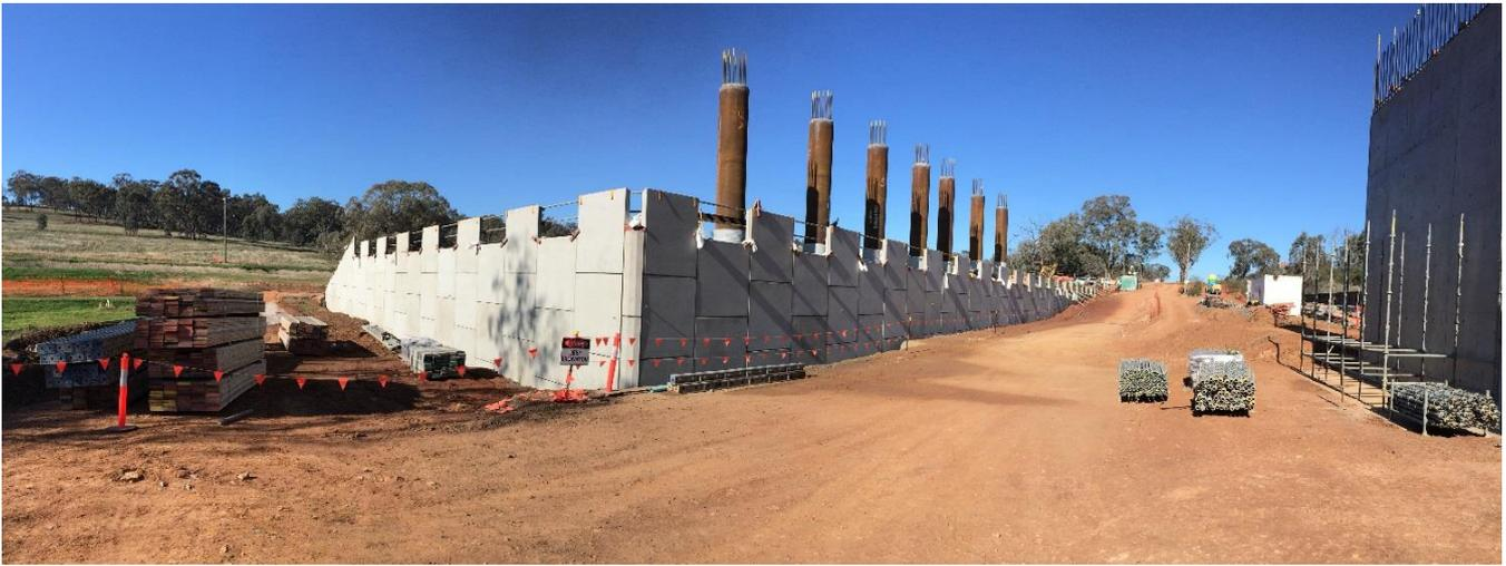
**Above:** Construction of the Reinforced Earth® bridge abutment walls begin.
