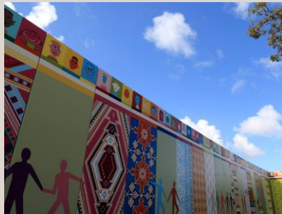
Above: Cantilevered Noise Wall – top part of the Reinforced Earth® retaining wall along Tonkin Highway on and off Ramps Above Right & Below: Redcliffe Park Wall at the Tonkin Highway/Dunreath Drive interchange, images courtesy of Gateway WA
