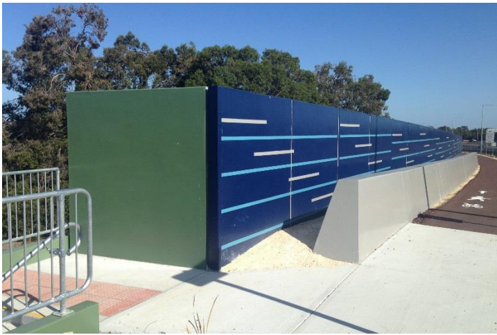
Above: Cantilevered Noise Wall – top part of the Reinforced Earth® retaining wall along Tonkin Highway on and off Ramps Above Right & Below: Redcliffe Park Wall at the Tonkin Highway/Dunreath Drive interchange, images courtesy of Gateway WA
