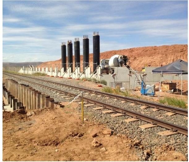
**Above Right:** Stabilizing the foundation soil by utilizing cement sand backfill.
