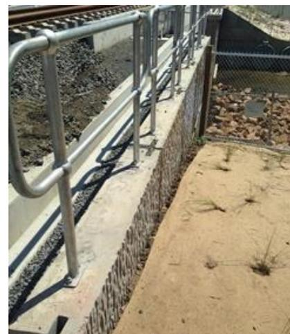
Main: Brady's Gully Under bridge Post and Panel wall
