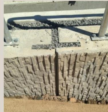
Above: The joints between the panels showing the recess where the support posts hide.
