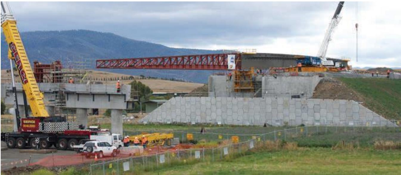
A bridge design involving a 70 metre bridge span was developed to avoid permanent impacts on the levee deposit. The long bridge span was launched from above rather than lifted from below to further protect the area. The Reinforced Earth® bridge abutment needed to be in place to allow the first girder of the long span to be launched from high above the levee. The first girder was then used to carry the remaining three girders across the levee.
