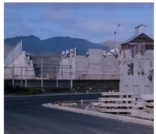
Main picture and top above: TerraClass® true abutment walls at the Blenheim Road Deviation Project in Christchurch
