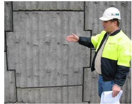
Left: Contractor John Holland engaged RECO to supply temporary TerraTrel® walls so that the construction of the TechSpan® tunnel and the permanent TerraClass® retaining walls could be staged to keep the Princes Highway open to traffic at all times. Above: RECO often develops a site-specific architectural finish, as was the case for the North Kiama Bypass.
