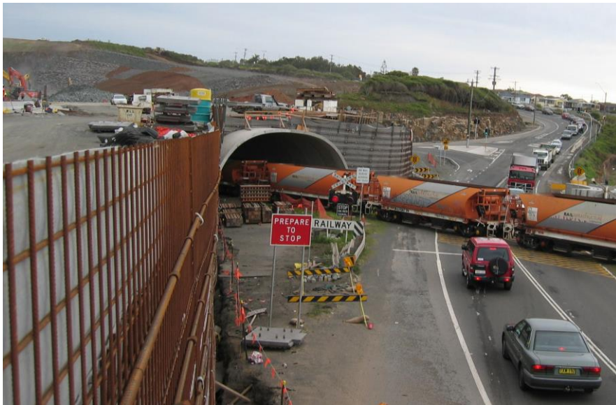
Left: Contractor John Holland engaged RECO to supply temporary TerraTrel® walls so that the construction of the TechSpan® tunnel and the permanent TerraClass® retaining walls could be staged to keep the Princes Highway open to traffic at all times. Above: RECO often develops a site-specific architectural finish, as was the case for the North Kiama Bypass.
