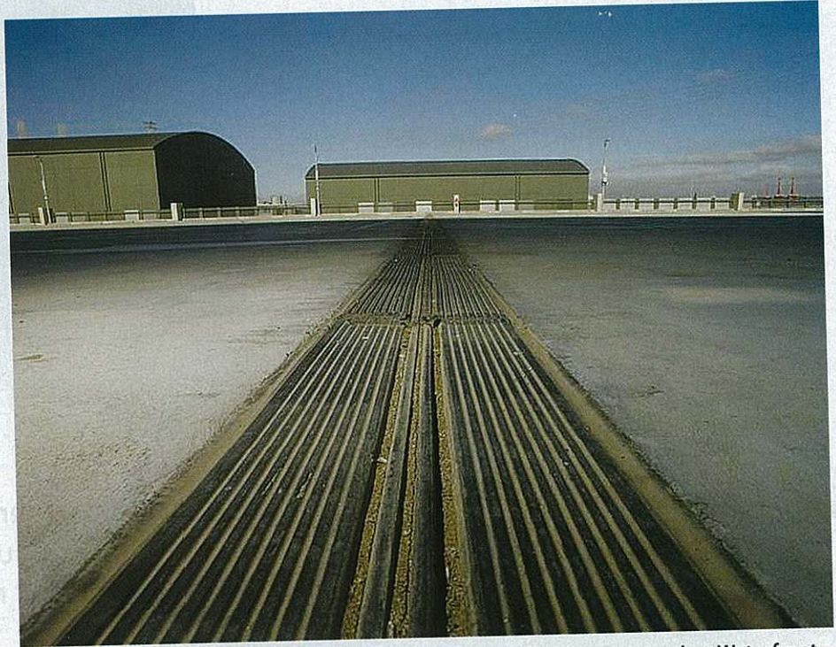
This high performance expansion joint was recently installed on a carpark at Waterfront City development in Melbourne's Docklands.
