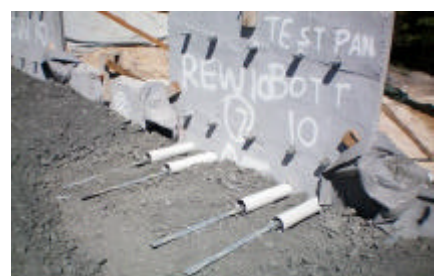
Main Picture: Installation of final TechSpan® unit.
