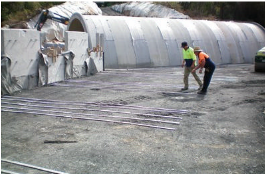
Left: Installation of REHas® soil reinforcing strips for the Reinforced Earth wing walls.
