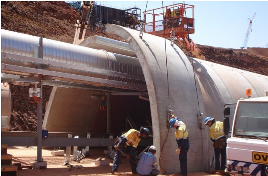
Left: TechSpan® precast arch unit is placed on the concrete footing.
