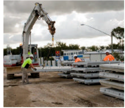
Left: Construction of Reinforced Earth abutments and retaining walls at Weakleys Drive Interchange.
