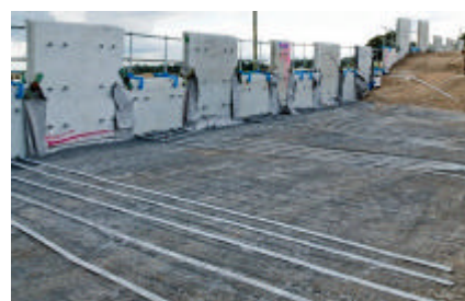
Main & Top: Horizontal rib panel finish. Above: REhas® galvanized steel reinforcing strips are unmatched for structural capacity and reliability.
