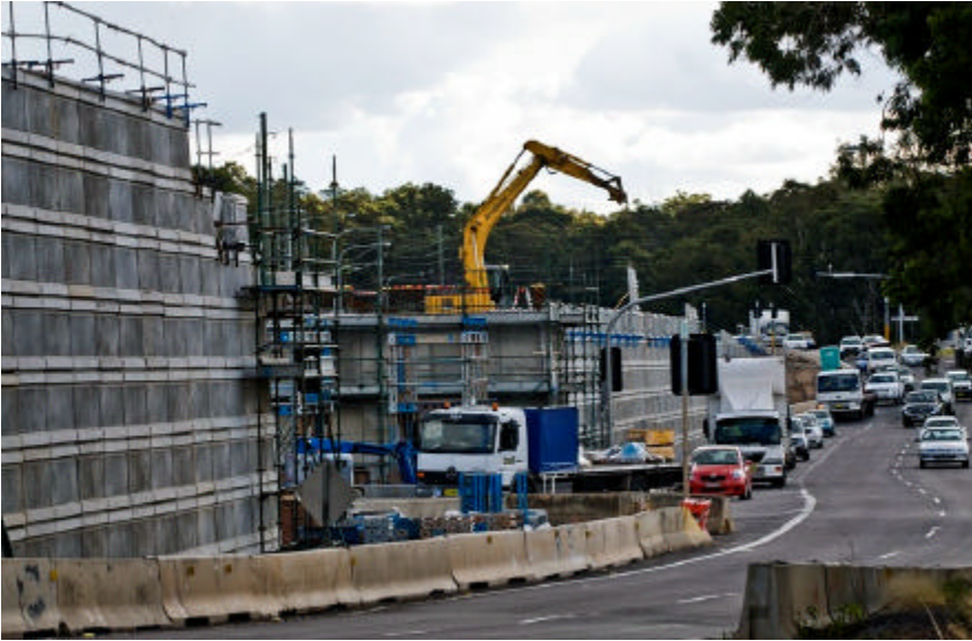
Left: Construction of Reinforced Earth abutments and retaining walls at Weakleys Drive Interchange.
