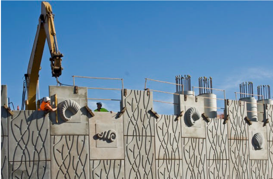
Left: Placing of TerraSet® Shell Pattern panel. Note checking of levels, and clamps ensuring correct panel alignment during construction.
