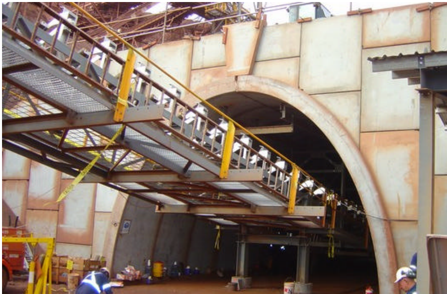
Left: Completed TechSpan® reclaim tunnel. Above: Installation of TechSpan® unit.
