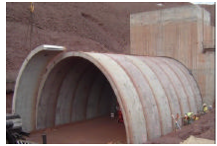
Left: Completed TechSpan® reclaim tunnel. Above: Installation of TechSpan® unit.
