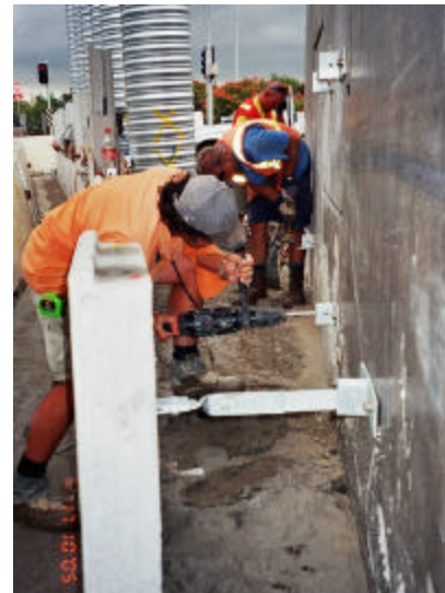
Main Picture: TerraClass® at Granard Road Duplication, March 2007. (After Upgrade)
