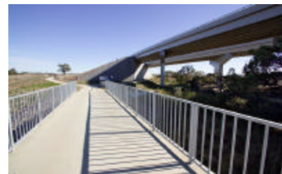
Merri Creek Bridges, Victoria
