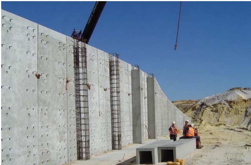
Left: Full height concrete channels, to be used as column formers. Above: Making up of panel moulds.
