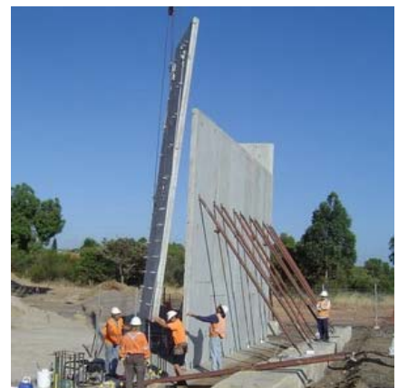
Main: TerraTilt® at Kwinana Freeway Interchange. Top: TerraTilt® at Karel Avenue Interchange. Center: TerraTilt® at South Street Interchange. Above: Installation of TerraTilt® panels.
