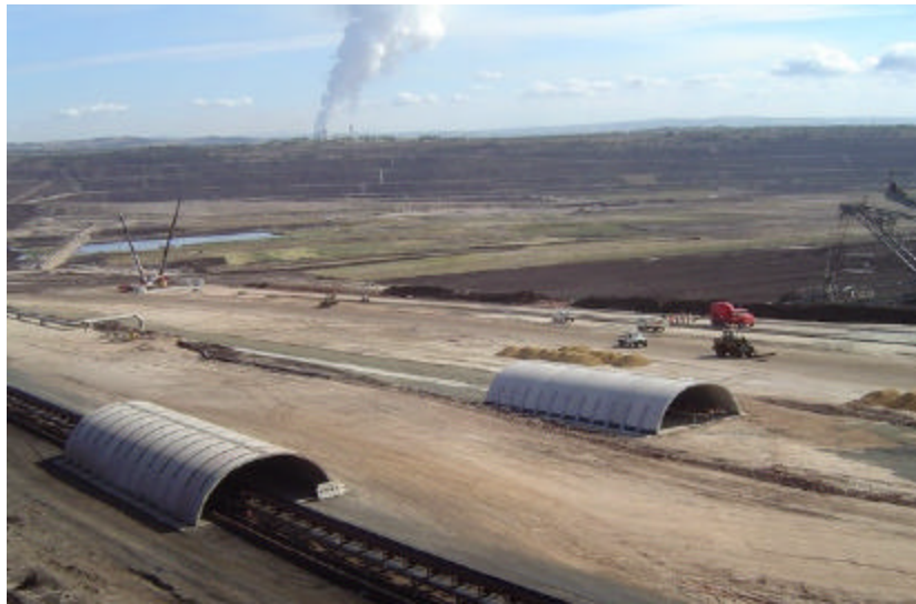
Left: Two of the Three Hazelwood Mine Conveyor TechSpan® Arches Above: Completed access road above TechSpan® Arches and conveyor.
