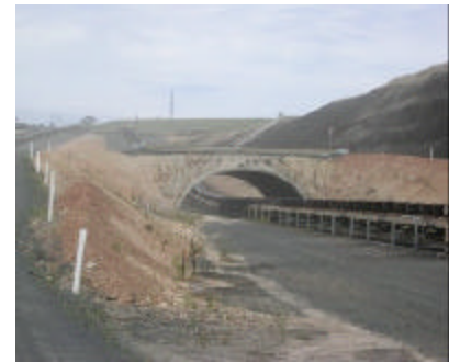
Left: Two of the Three Hazelwood Mine Conveyor TechSpan® Arches Above: Completed access road above TechSpan® Arches and conveyor.
