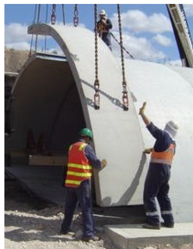
TechSpan® Arch construction at Hazelwood Mine
