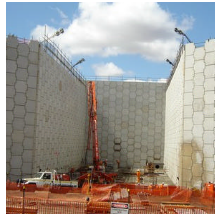
Left: Aerial Photograph Above: Installation of final course of TerraClass® panels
