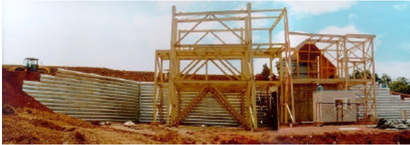
Left: Sepon Gold. Dump Structure and Primary Crusher Construction
