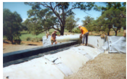
Main Picture: Saturday 16h00: TechSpan® Arch Tunnel erection completed.
