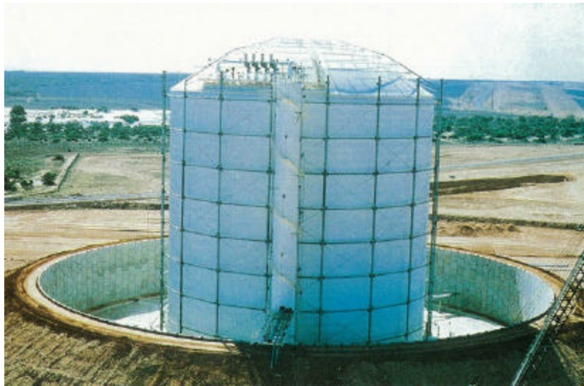
Left: Close up view of 10.5m high, 75m-diameter containment dyke. Above: Cross section of the structure.
